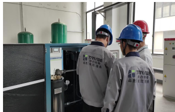
Machine appearance inspection
